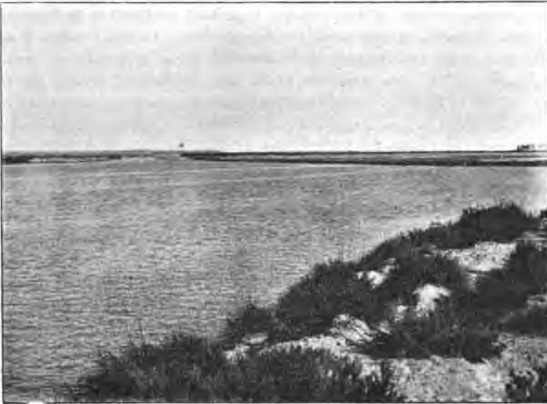
HELMAND RIVER AT KUHAK, SHOWING MOUTH OF THE ROD-I-SEISTAN AND THE BAND-I-SEISTAN WEIR.
