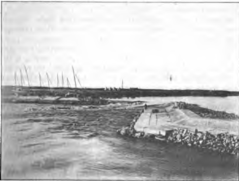
FIG. 2.—BROKEN BARRAGE AT MOUTH OF HINDIYE CANAL, 5 MILES BELOW MUSSEYIB. TO THE LEFT, HINDIYE; TO THE RIGHT, EUPHRATES, LOOKING NORTH-WEST.
